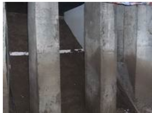
图 3 试验槽与抗滑桩的施工照片 Fig.3 Picture of test flume and anti-slide
